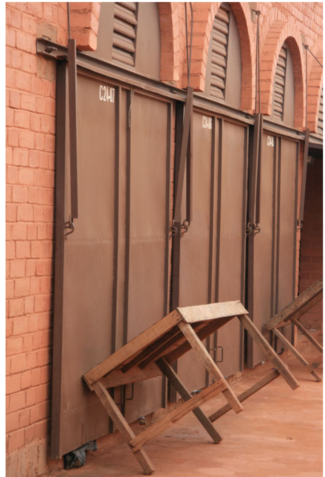
9.29 The steel, up-and-over doors-cum-awnings of the market of Koudougou. Photograph Belinda van Buiten
