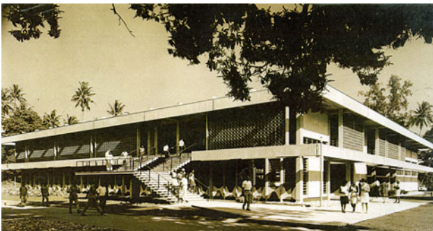
14.22 National Library in Dar es Salaam by Almeida in 1968. Source Anthony Almeida
