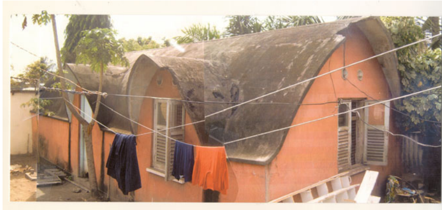
8.3 A 'parabolic' house in Dar es Salaam. This house is strongly reminiscent of the prefabricated concrete houses developed by Ernst May for East Africa. This unique house has since been demolished. Sophie Hayen and Sophie Lemmens
