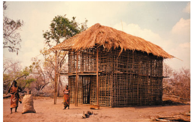
6.4 Charcoal burner's house under construction in the wilderness of southern Tanzania, 1988
