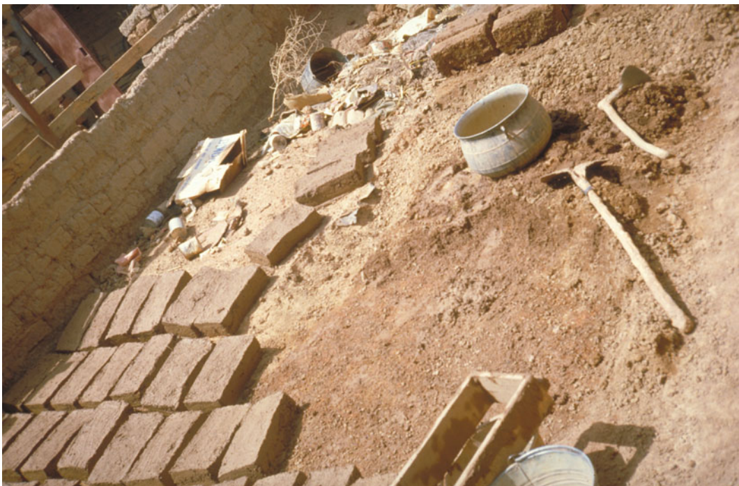
9.10 The modernizing of Larlé-Extension in the 1980s. The banco of the informal Larlé is pulverized, mixed with water and straw and reused in new residences
