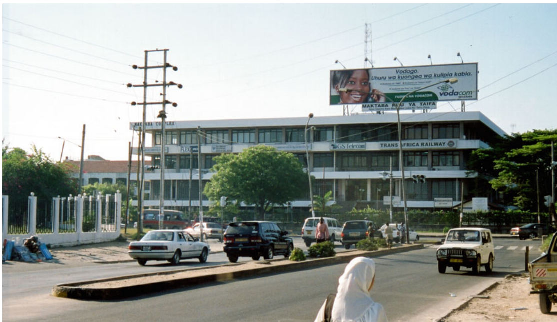
14.24 National Library by Almeida in 2000. Almeida took account in his design of a vertical extension. It was increasingly difficult in the 1990s for the library to remain functioning, and it was decided to entrust the extension to a commercial developer in order to guarantee the survival of the library. But this meant that no account was taken of Almeida's design. Photograph Antoni Folkers
