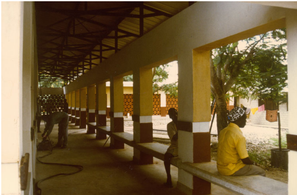
12.11 Renewed wards at Turiani Hospital at the end of the 1990s
