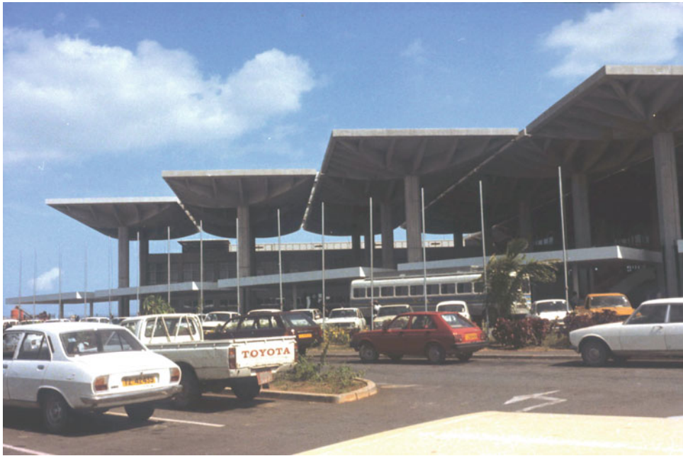
7.27 The terminal building of Dar es Salaam International Airport by Paul Andreu, early 1980s. Inverted umbrella roofs, discharging the rain water through the columns
