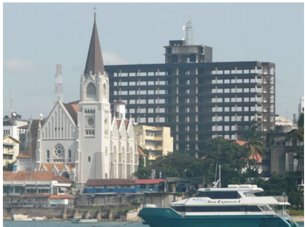
16.6 The restored St. Joseph's Cathedral in the quickly changing urban context of Dar es Salaam
