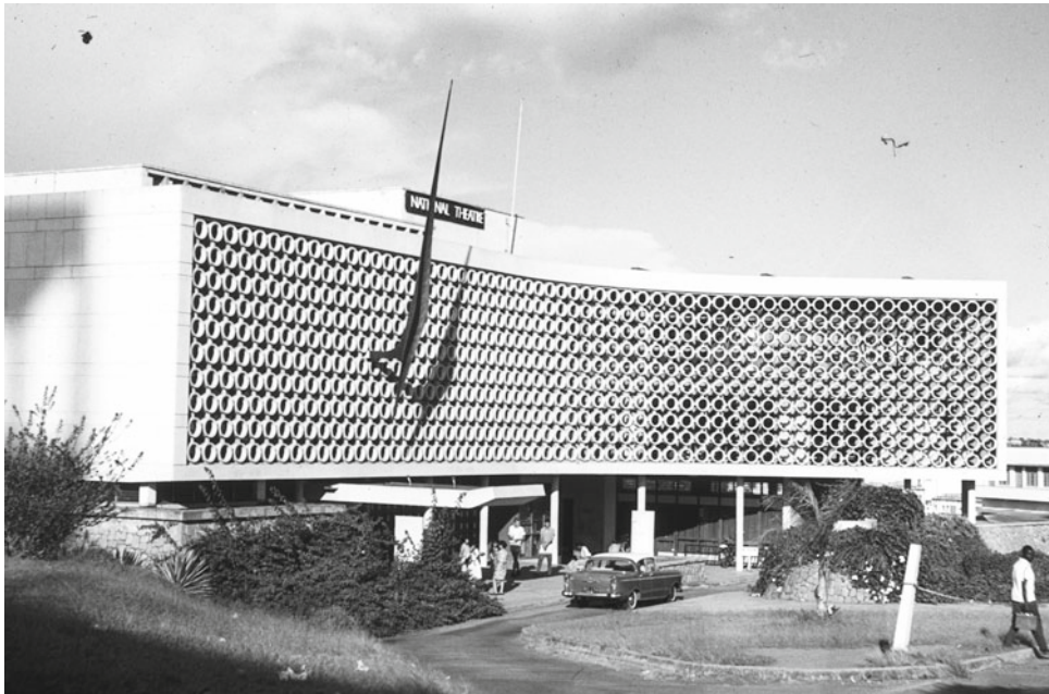
10.28 The National Theatre in Kampala by Peatfield & Bodgener. Source Georg Lipsmeier
