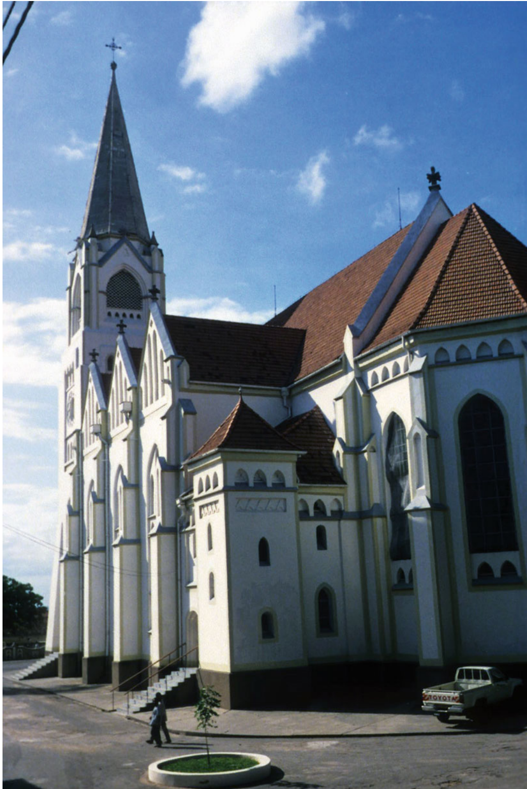
16.1 St. Joseph's Cathedral before restoration (see also p. 53). Source Georg Lippsmeier
