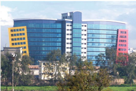
9.3 The renovation of the former Nasaco building in Dar es Salaam by Nuru Inyangete and Kayzi Kalambo in 2002. Photo Nuru Inyangete
