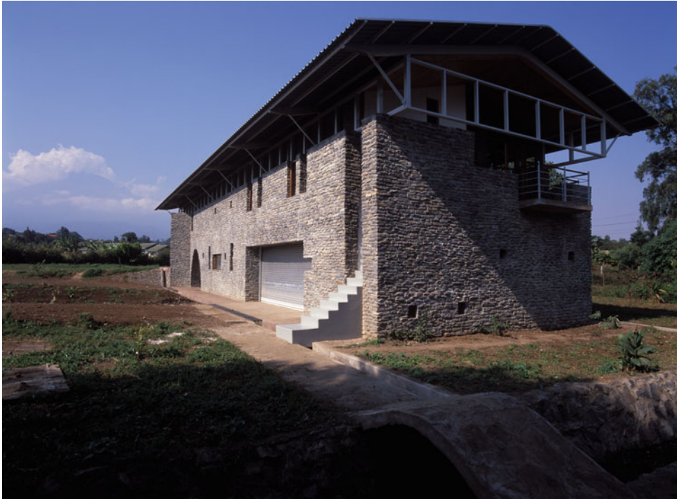
9.37 Van der Wel House in Arusha. The house is earthquake-resistant and built of locally obtained limestone with 60 cm thick walls and a cantilevered Vierendeel girder serving simultaneously as a continuous band of clerestory windows. Photograph Nick Parfitt
