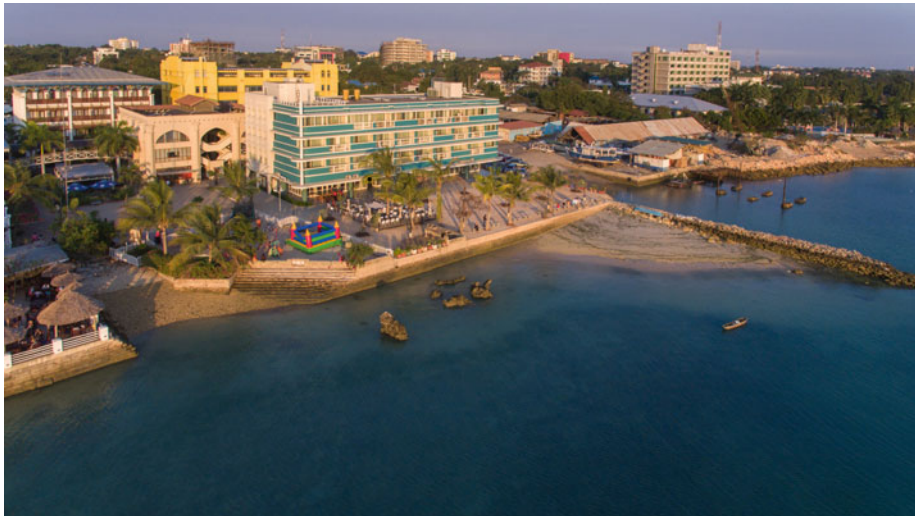
11.18 Waterfront of Slipway, 2017
