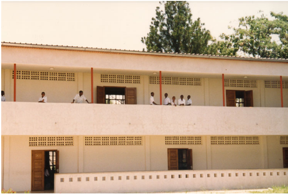
10.31 The rehabilitation and extension of the School for the Deaf in Tabora in the 1990s
