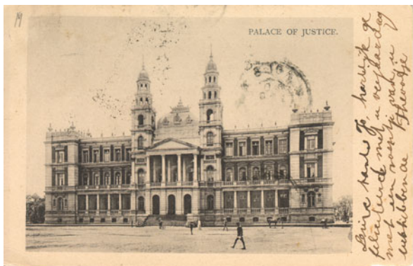
14.17 Pretoria High Court by Wiarda (circa 1890). 'Boer baroque' according to Braam de Villiers
