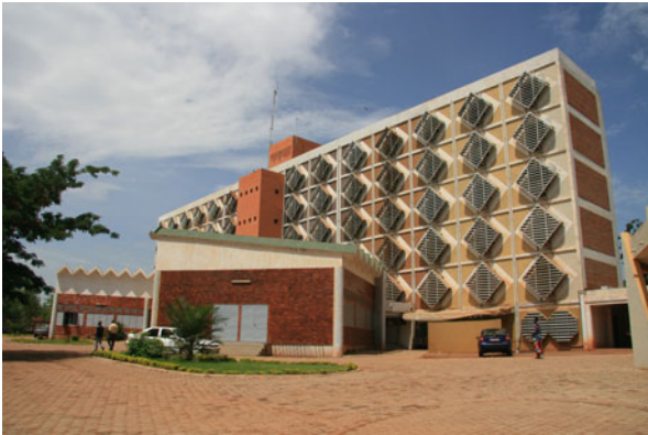
18.4 Ministère des Finances in Ouagadougou in 2008. A new screen facade has been placed in front of the rigid modernist walls hiding the air-conditioning system. Photograph Belinda van Buiten
