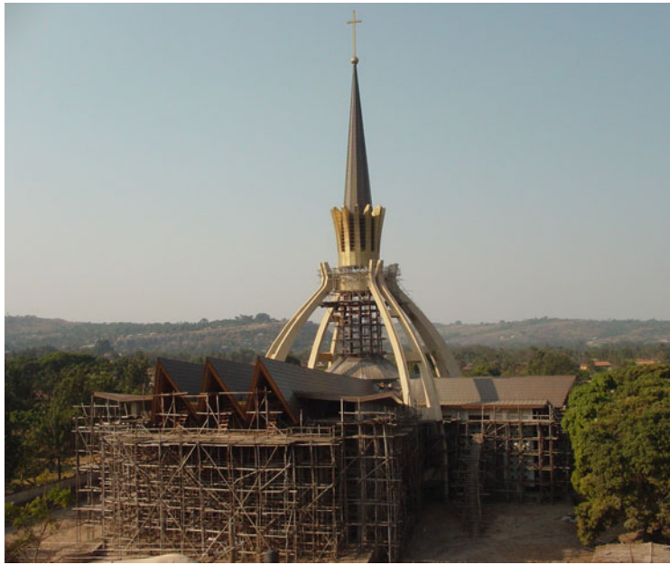
17.12 The construction site in 2009. Photograph Rudi van Winkelhof
