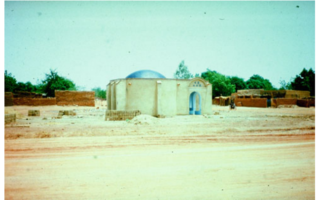
8.17 The DGUT field office on completion in 1984
