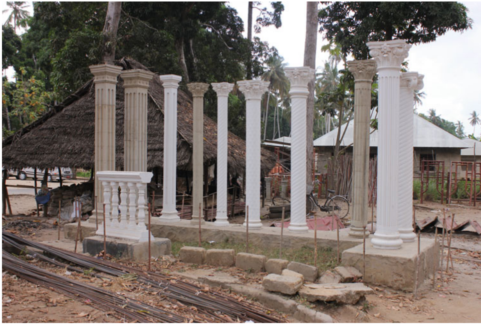
9.17 Prefabrication of concrete classical columns and capitals on Zanzibar. Photograph Antoni Folkers
