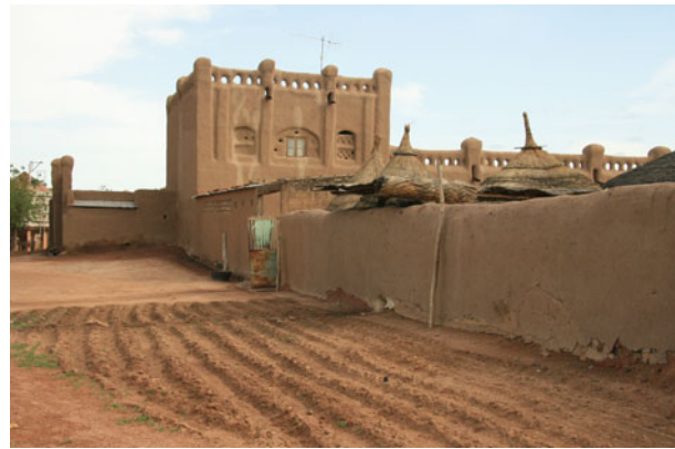
18.12 The Na-yiri in Kokologho. It is said that this palace of the local Chef Coutumier was designed by a French missionary. The central part with one story betrays a French interpretation of the traditional monumental mud architecture which transformed Ouagadougou into a Bancoville in the early colonial period. [See also illustrations on p. 103 middle] Photograph Belinda van Buiten
