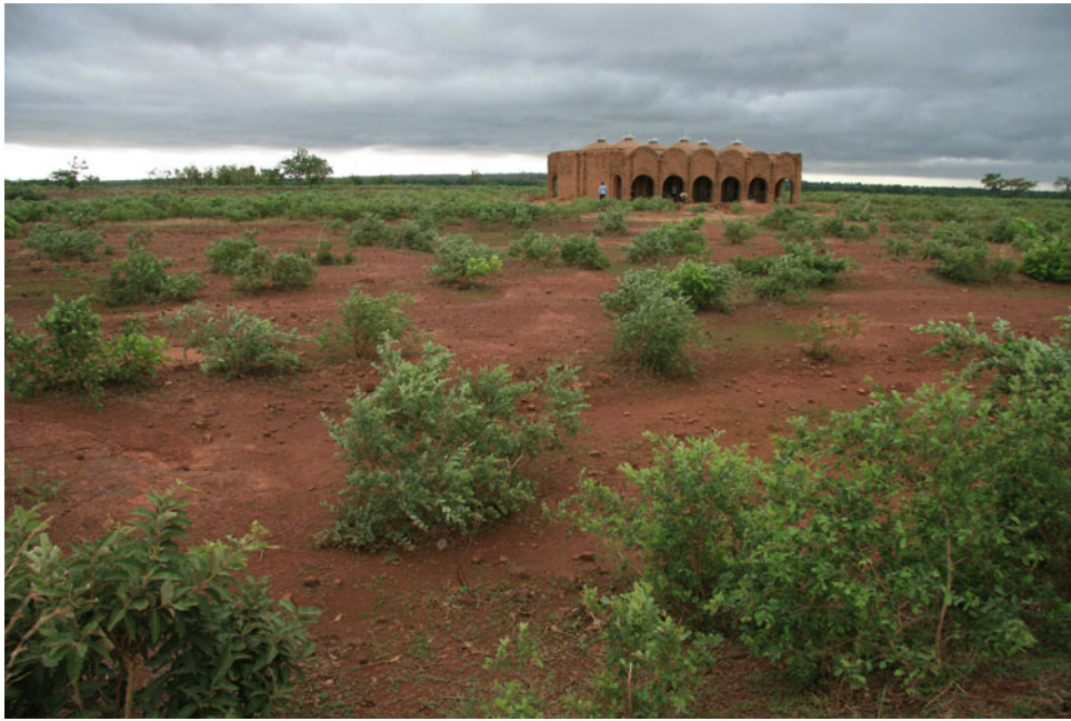
9.19 A school building near Réo in Burkina Faso in 2008. The building, developed with Swiss help and planning, was at that moment neither complete nor in use yet it was already a ruin. Photograph Belinda van Buiten
