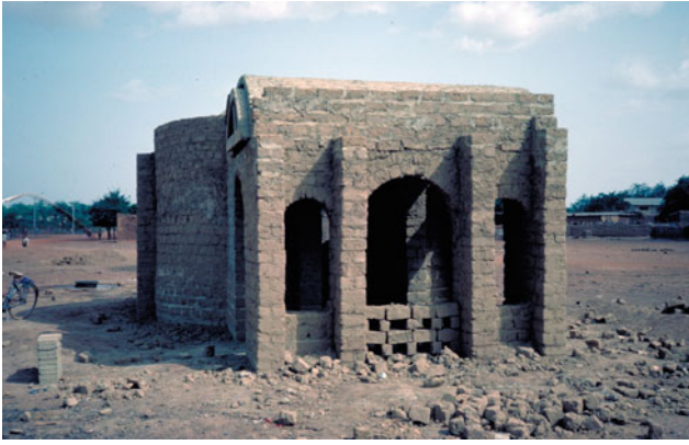
8.16 The completed structural shell of the DGUT field office
