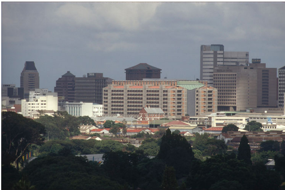
13.4 Eastgate building in Harare by Mick Pearce. This great office block uses half the energy of a conventional building because of the ingenious ventilation system that was inspired by a termite-heap. Photos David Brazier
