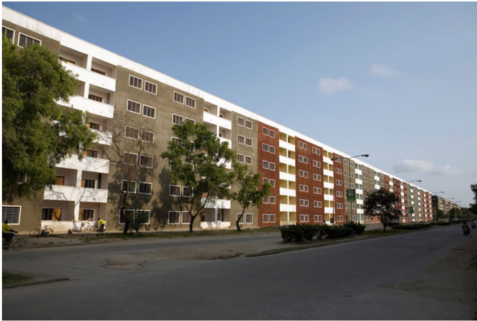
3.54 New building in Michenzani in 2008. Photograph Mieke Woestenburg
