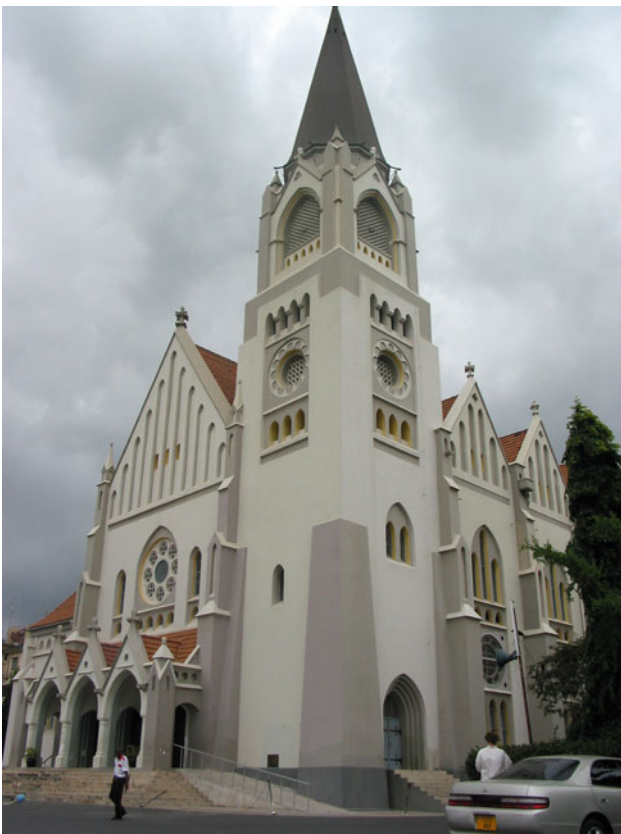
16.5 St. Joseph's Cathedral after restoration. Photograph Belinda van Buiten
