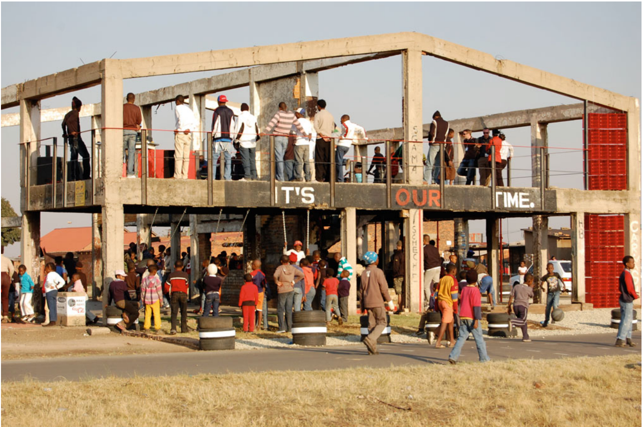
9.2 Mashinini Beer Hall in the Kwa-Thema project in Johannesburg by Hannah Leroux and students of the University of Witwatersrand. A community building in the Kwa-Thema project, burnt to the ground during the 1976 township riots, was subsequently reclaimed and rebuilt by the inhabitants. Photograph Hannah Leroux. See also the cover photo
