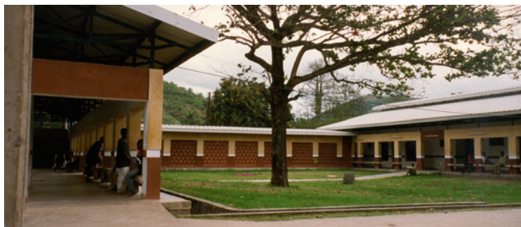
12.5 Renewed wards at Turiani Hospital at the end of the 1990s
